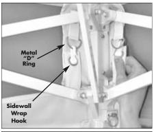
**Step 2.** Locate desired front entry point. Starting from the inside right corner, hook the sidewall wrap onto the metal D-rings that are located on the corners of frame. Continue hooking the sidewall wrap to metal D-rings on the outer side of the trusses until sidewall wrap is completely hung around remaining three corners.
